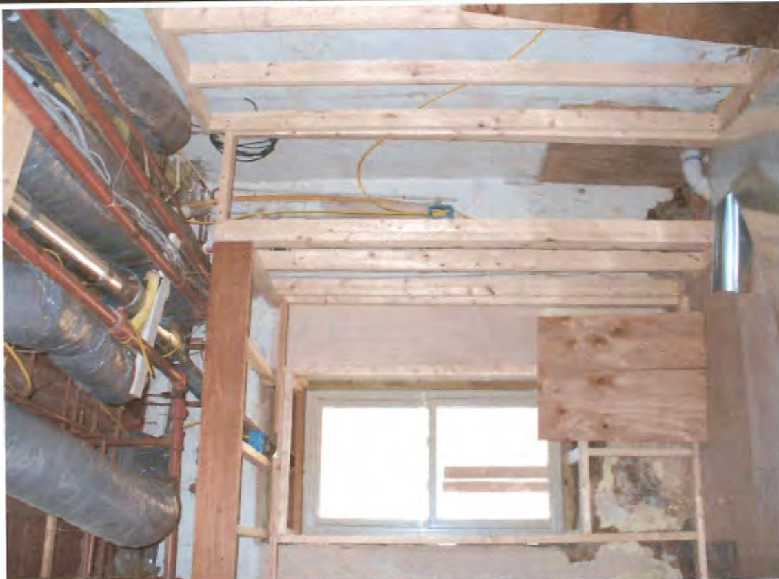
19 OFFICE: BASEMENT APARTMENTS CONSTRUCTION
