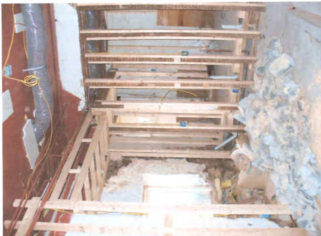
20 OFFICE: BASEMENT APARTMENTS CONSTRUCTION
