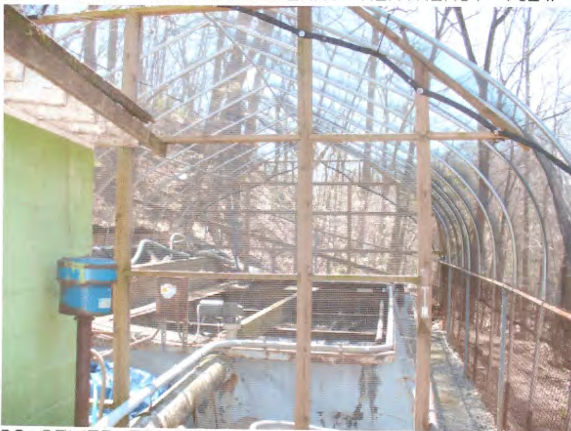
28 SEWER TREATMENT PLANT: SOUTH VIEW
