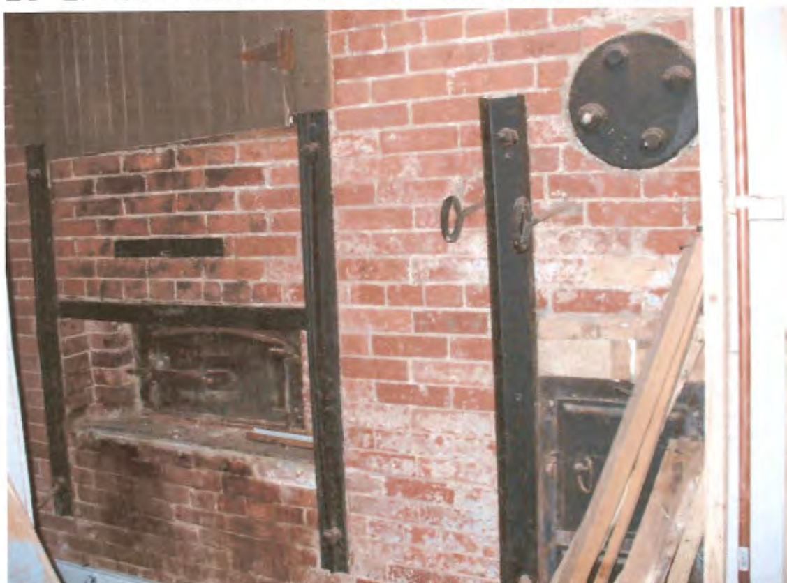
24 OFFICE: BASEMENT CAST IRON STOVE
