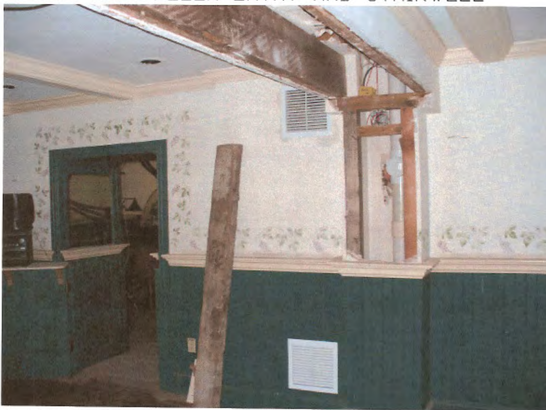
8 INN: BASEMENT ROOM
