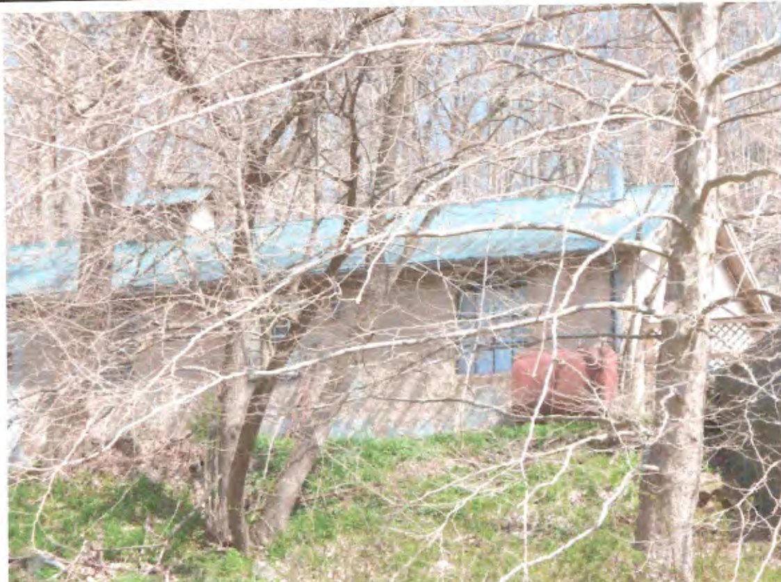
45 CONCRETE BUILDING: AST
