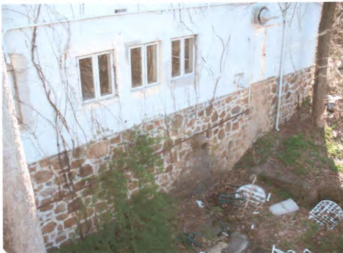
2 INN: SOUTH END REAR WALL
