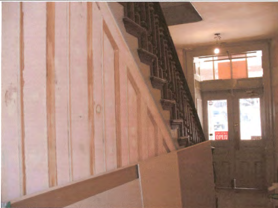
7 INN: MAIN FLOOR ENTRY AND STAIRWELL
