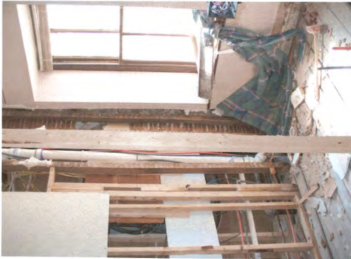
4 INN: UPPER LEVEL ROOMS BEING REMODELED
