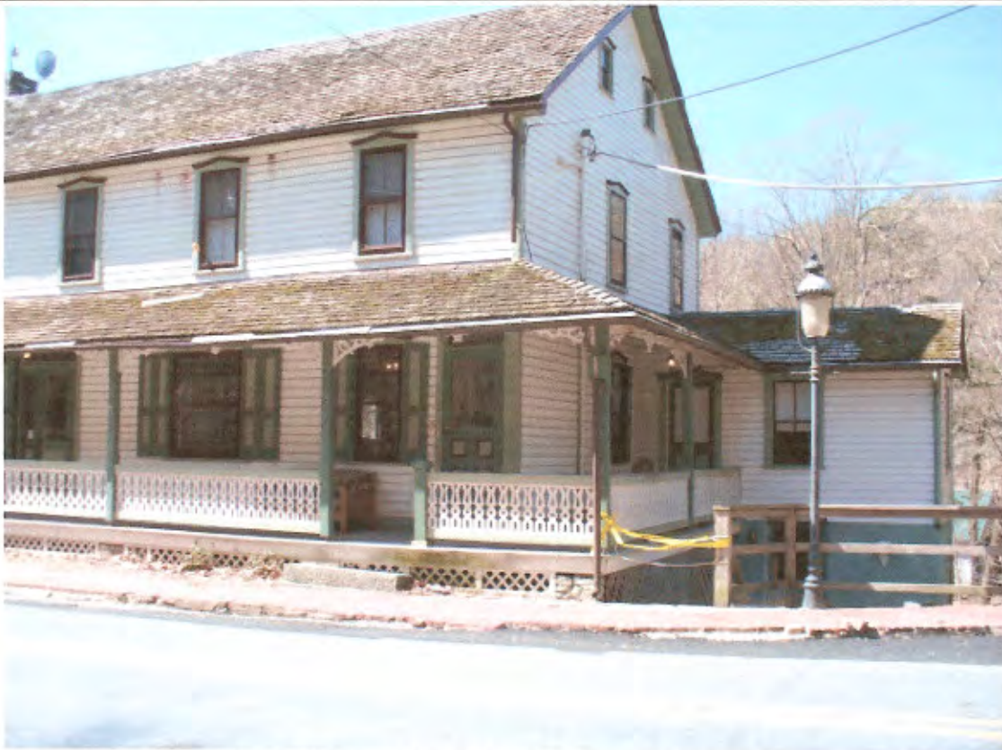
15 OFFICE: FRONT VIEW (FORMER GENERAL STORE)
