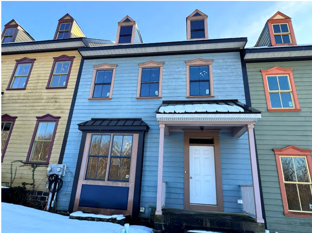
The Falls at Saint Peters (24 Falls Drive) Lot 15 Existing Unfinished Interior Townhouse Unit
