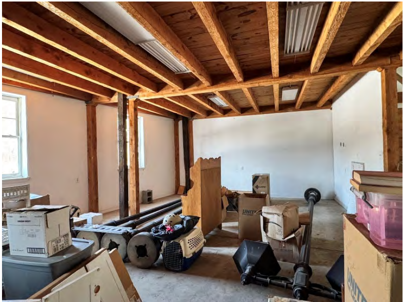
Vacant – Building 3260 Saint Peters Road
